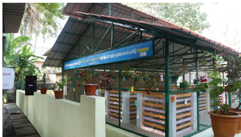
Image: Garbage heaps at overburdened MCF - Mangalapuram GP, Thiruvananthapuram
